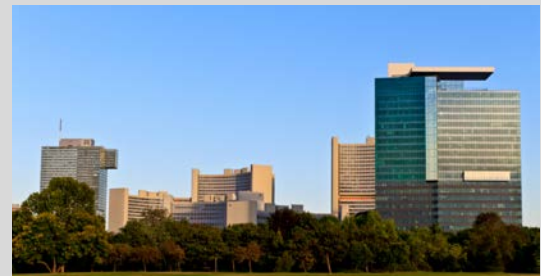
PROJECT // ACV - AUSTRIA CENTER VIENNA
