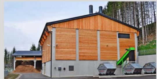
PROJECT // HEATING PLANT MARIAZELL
