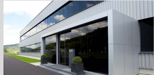
PROJECT // PRODUCTION HALL LIST COMPONENTS & FURNITURE GMBH EDLITZ-THOMASBERG
