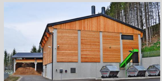
PROJECT // HEATING PLANT MARIAZELL
