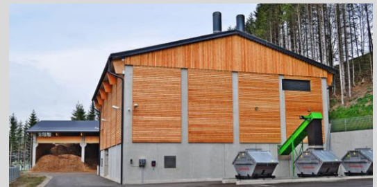
PROJECT // HEATING PLANT MARIAZELL
