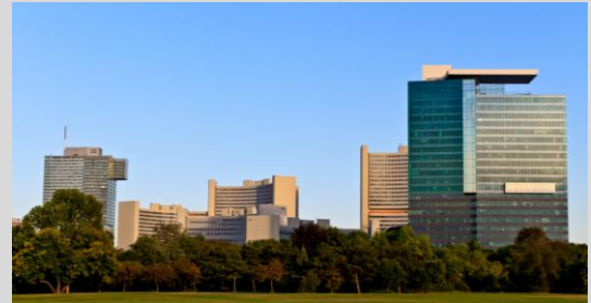
PROJECT // ACV - AUSTRIA CENTER VIENNA
